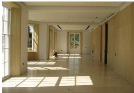
Site Photo: Sash windows, Haywood Green Farm
