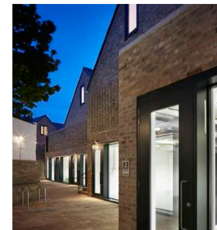
Photo: Fig. 3, Courtyard, Foundry Mews, Barnes
