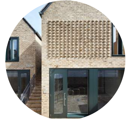
^ Office Entrance, Foundry Mews, Barnes
