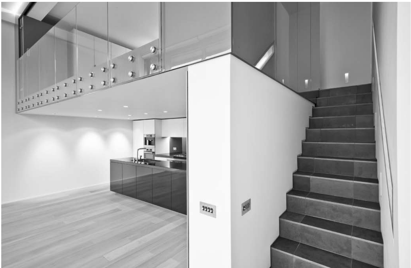
Detail of flush handrail Corner shadow gap Staircase and Mezzanine, Gallery Lofts, London
