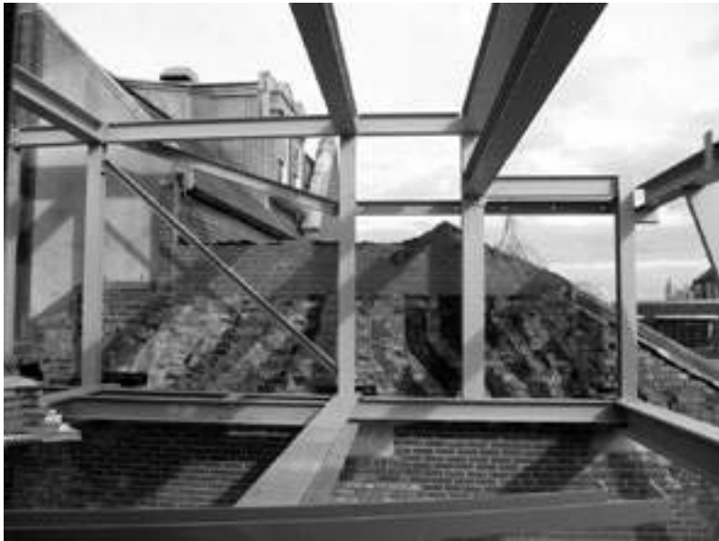
EASTERN STEEL FRAME AND HISTORIC PARTY WALL FLUES
