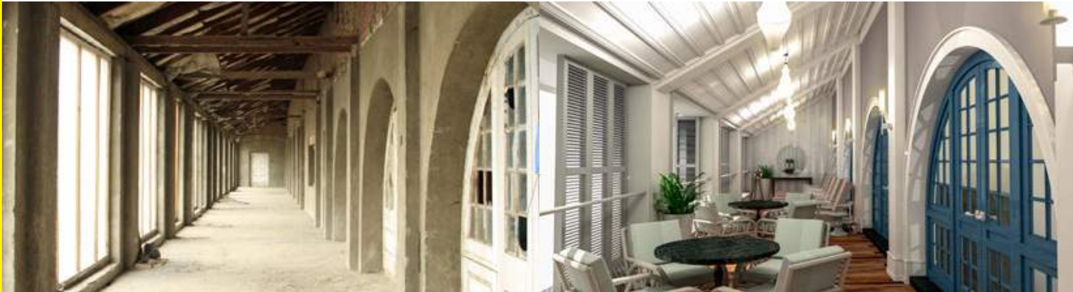
PHOTOGRAPH: EXISTING VERANDA
